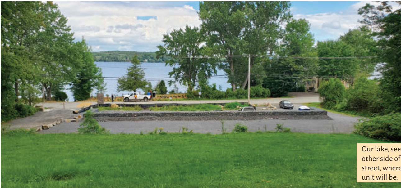
Location of the future sanitary unit.
